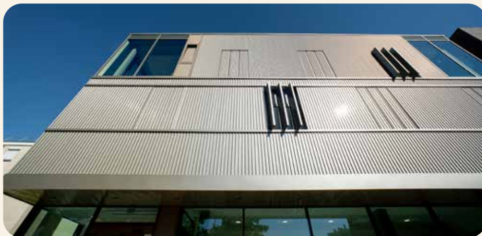
Medical Centre Orly, France Insulated Panels JI Sonora; JI Brise; JI Albe
