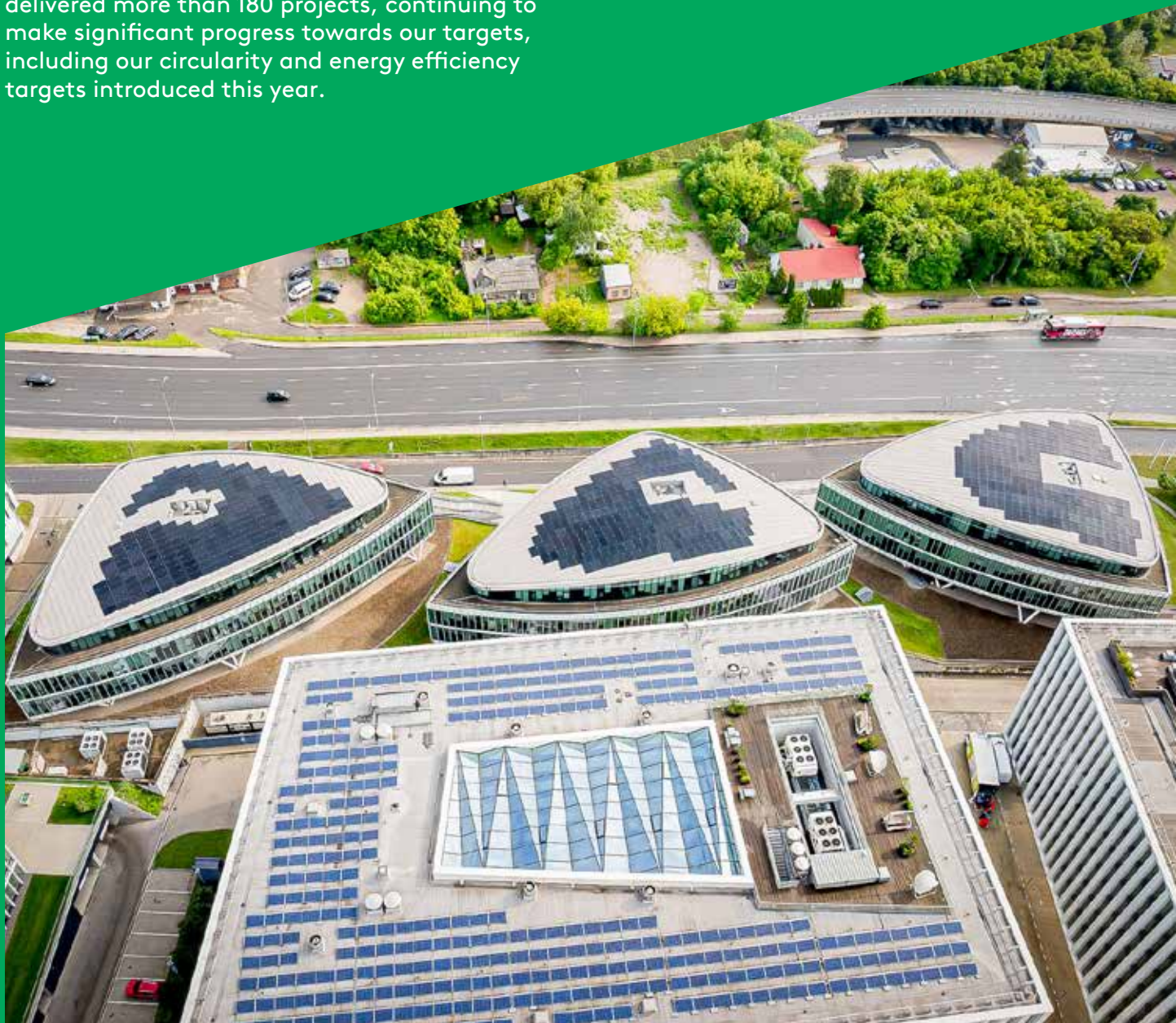
BALTIC HEARTS OFFICES ..... Vilnius, Lithuania Insulated Building Envelopes Dome Solar roof-solar PVC
